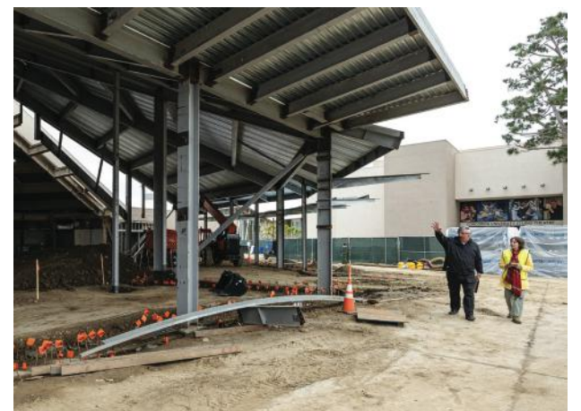
PICTURED ABOVE: Tim Odle leads a tour around the construction site
