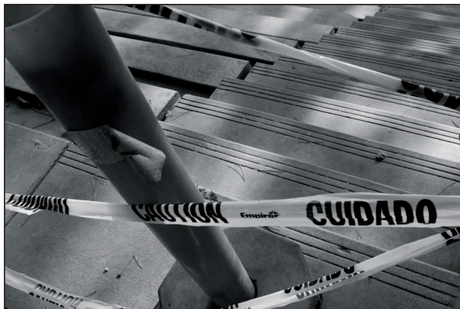
Due to tree roots and other causes, paved walkways like the steps of the Outdoor Amphitheatre are being repaired, forcing students to find alternate routes to classes.
